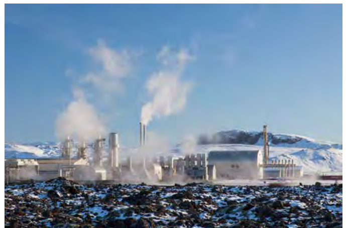
Taken on February 16, 2016, this photo depicts the Svartsengi Power Station, a geothermal power plant in the Svartsengi geothermal field near Grindavik, Iceland. (Photo by: Arterra/Universal Images Group via Getty Images)
